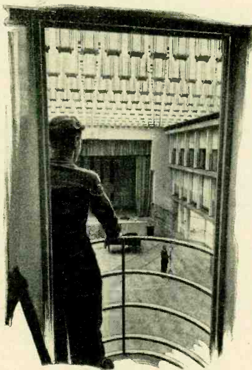
THE MAN ON THE BRIDGE. A photograph taken from the centre of the moving wall in the Hamburg studio. By advancing or withdrawing the wall it is possible to alter the studio acoustics to suit different types of programme.
